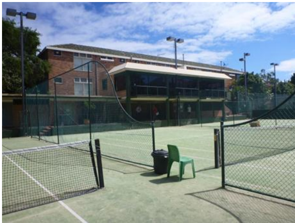
PICTURE 3 – EXISTING CLUB BUILDING WITHIN THE SITE
